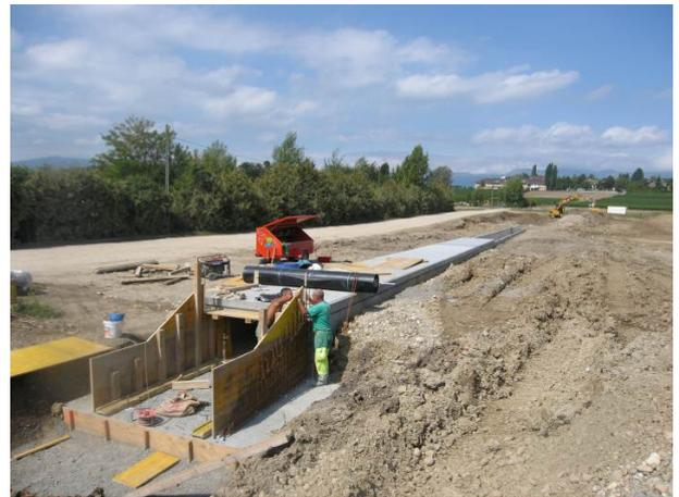
Figure 24 Construction dalot
